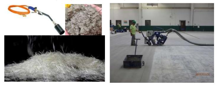
When the fiber is not burned off the surface, the fiber will stick up above the concrete surface and wick the moisture from the slab.
