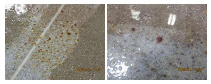
The photos above are of a moisture failure due to the concrete fibers not being properly covered/coated with moisture reduction barrier (MRB). The failure happened within days after installation of the MRB. The floor was not properly burned prior to the installation. The floor required 100% grinding of the MRB, shot blasting, & fiber burning at a cost of over \$80,000
